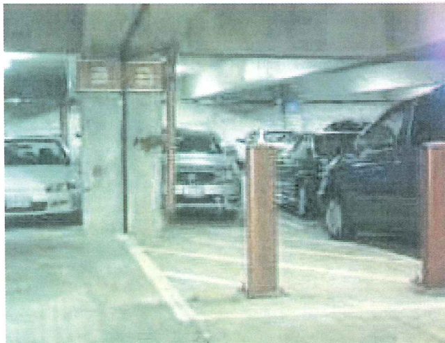
(Fig. 4.9) Bollards and striping to create an access path in a parking garage. Bright signs at the top of column help to locate the valve.
