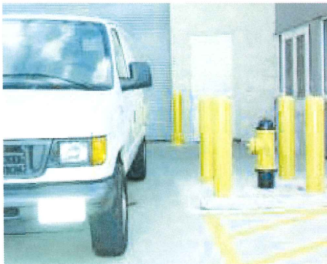
(Fig. 2.14) This hydrant should not have been located where it is likely to be blocked. Loading docks, by nature, will likely have vehicles parked. This is an example of building a potential deficiency into a facility. The truck could prevent use of the large pumper connection or cause the base to be kinked when used. Note the yellow bollards which protect the hydrant from vehicle collision.
