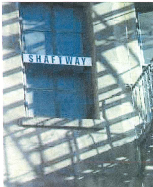
(Fig. 2.26) Exterior shaftway marking.
