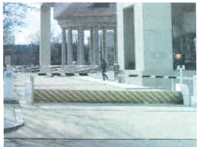
(Fig. 2.10) Pop-up barricades such as these are appearing more frequently due to security concerns. Unless security forces are constantly present to operate them, however, the fire department should be provided with a means to do so.
