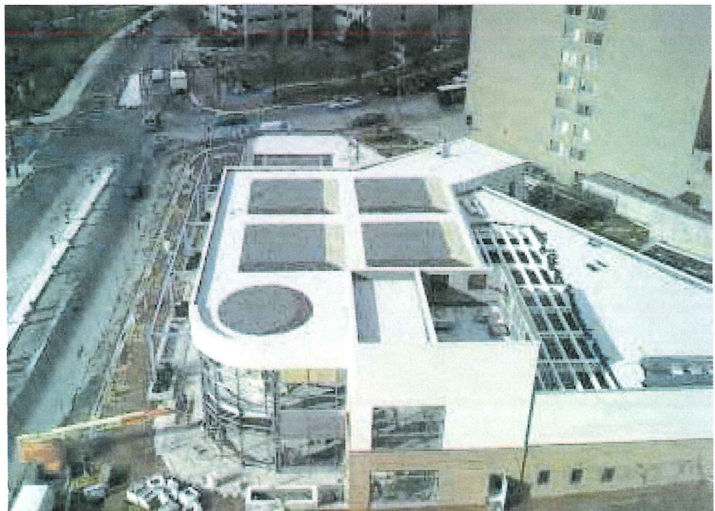
(Fig. 2.3) A combination of two public roads and two private fire lanes provides full perimeter access to this building.
