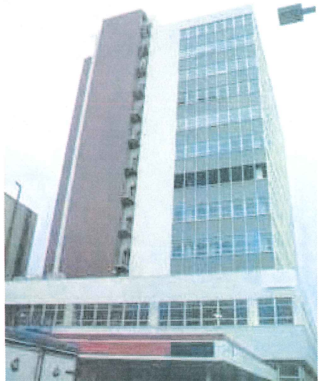
(Fig. 4.5) Exterior view of open air vestibules between the stair and the interior of a building.
