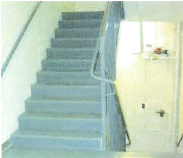
(Fig. 4.2) Hose connection on intermediate landing as viewed from the main landing where the stair entry door is located.
